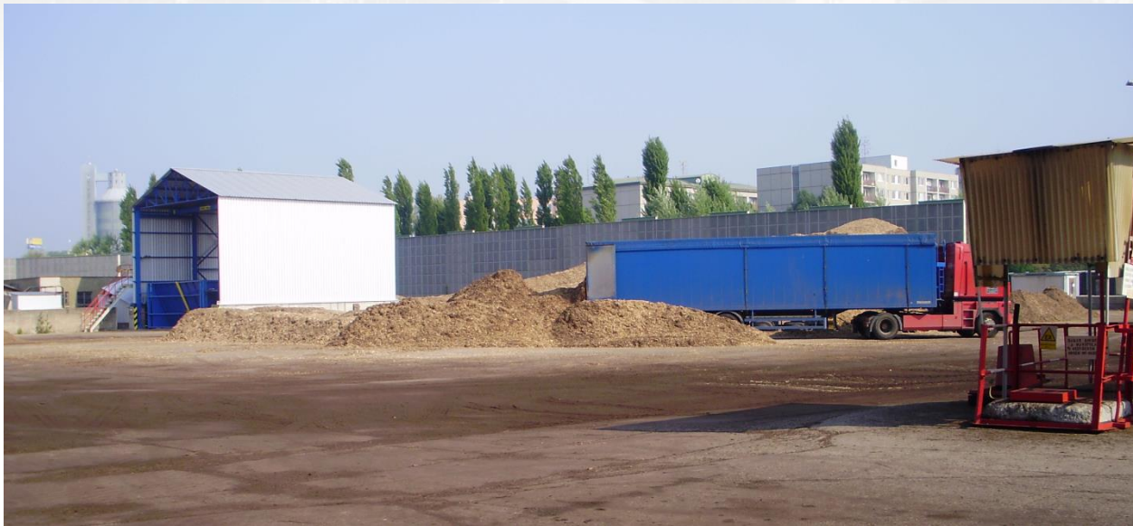
Biomass unloading yard
