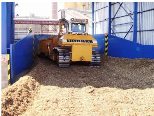
Biomass receiving area with underground screw
